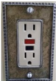
Ground Fault Circuit Interrupters (G.F.C.I.)
