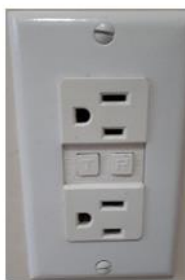
Ground Fault Circuit Interrupters (G.F.C.I.)
