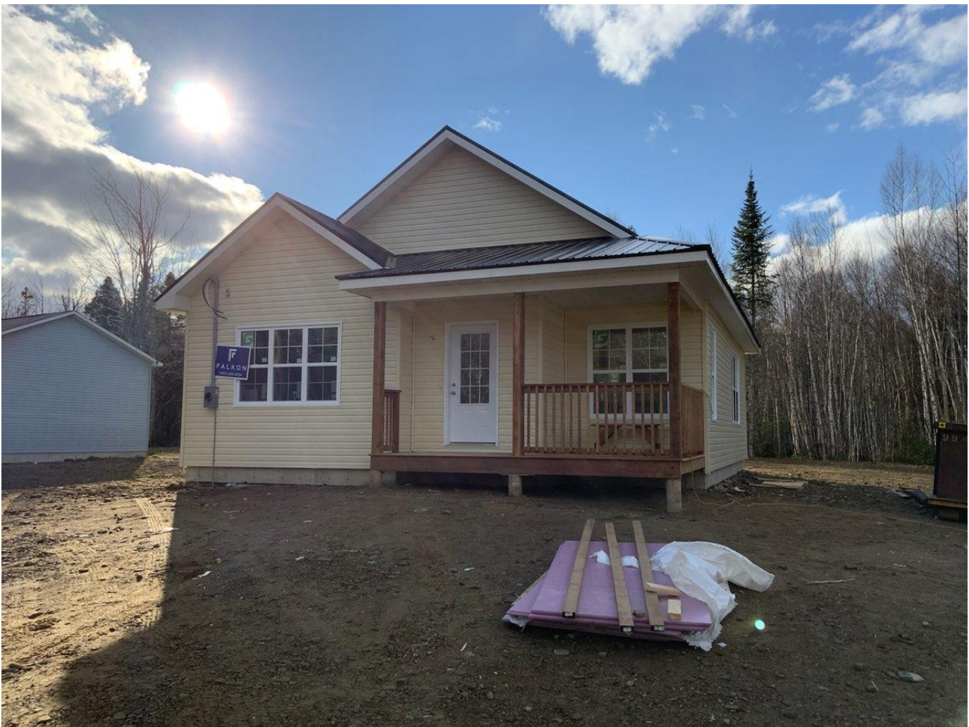
Exterior of the Esgenoopetij house build
