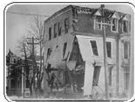
This photo shows two of the hundreds of damaged buildings after the explosion.
